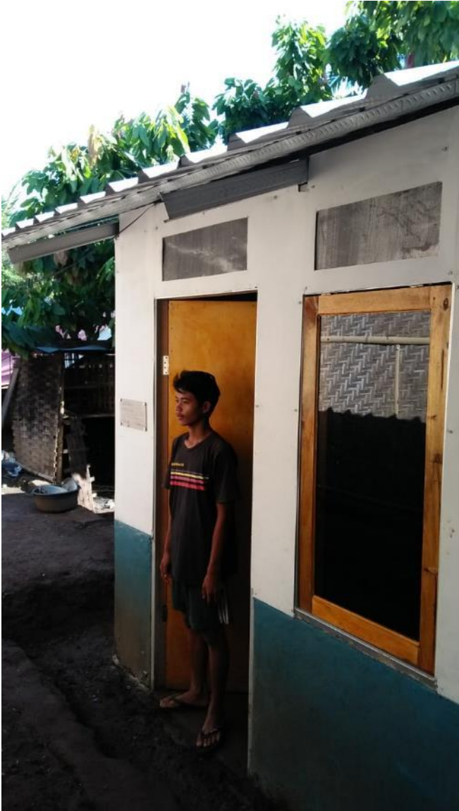
House condition AFTER intervention with temporary shelter assistance.
