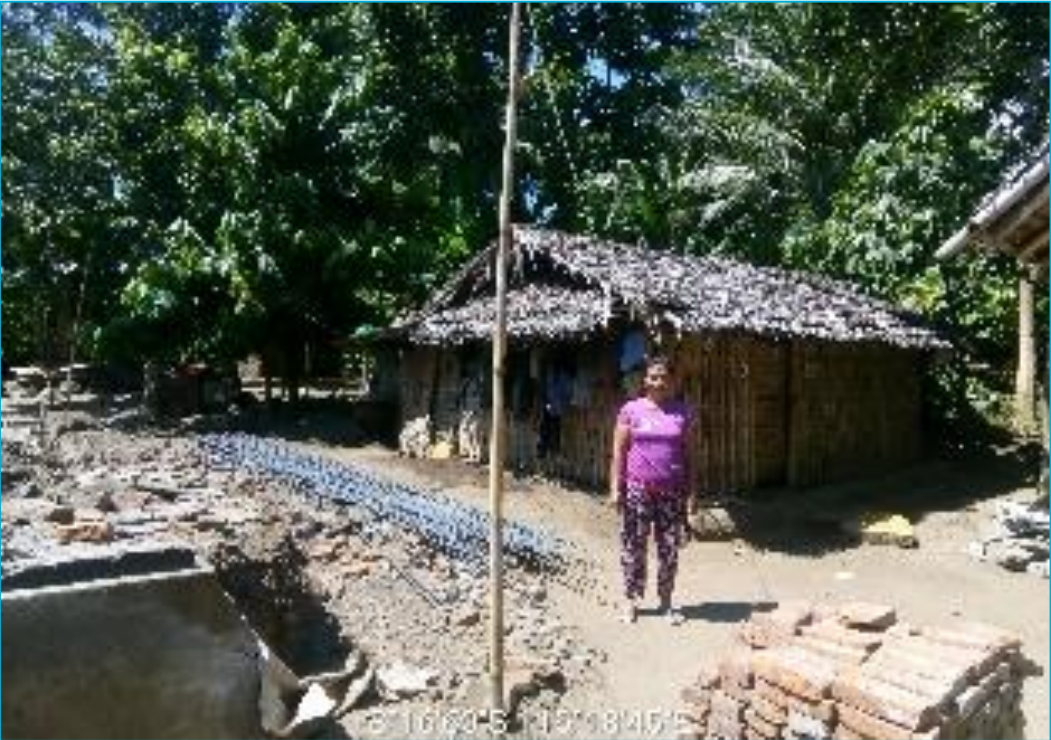
House condition BEFORE intervention
