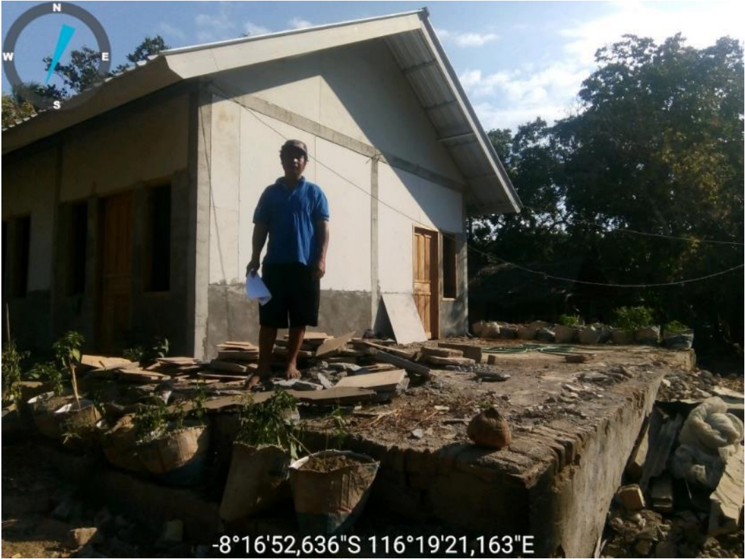
House condition BEFORE intervention
