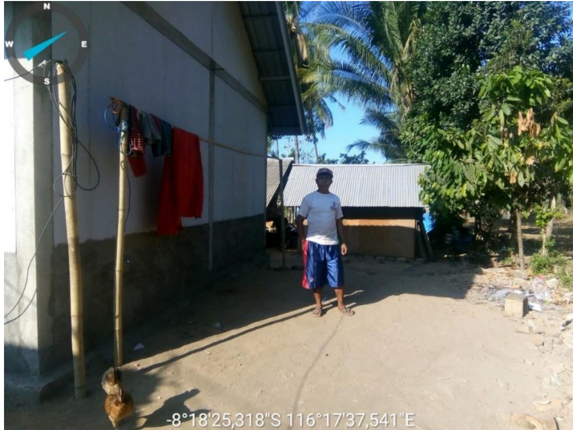
House condition BEFORE intervention
