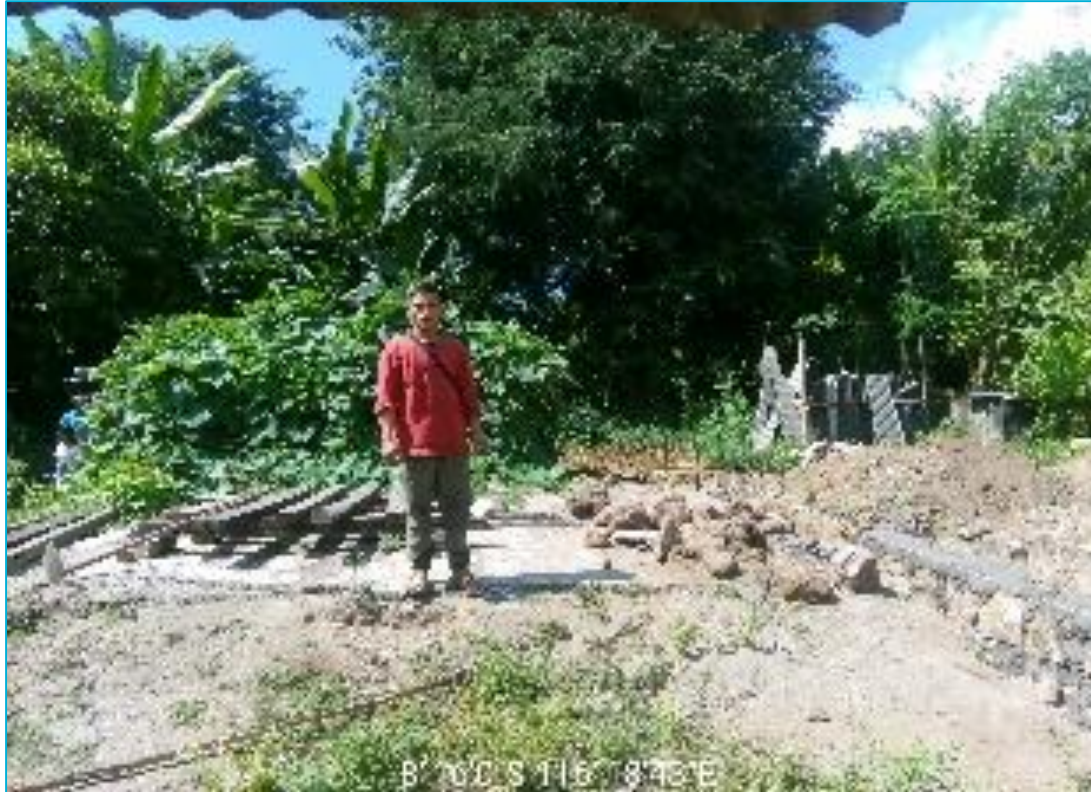
House condition BEFORE intervention
