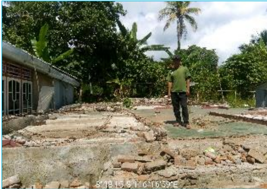
House condition BEFORE intervention
