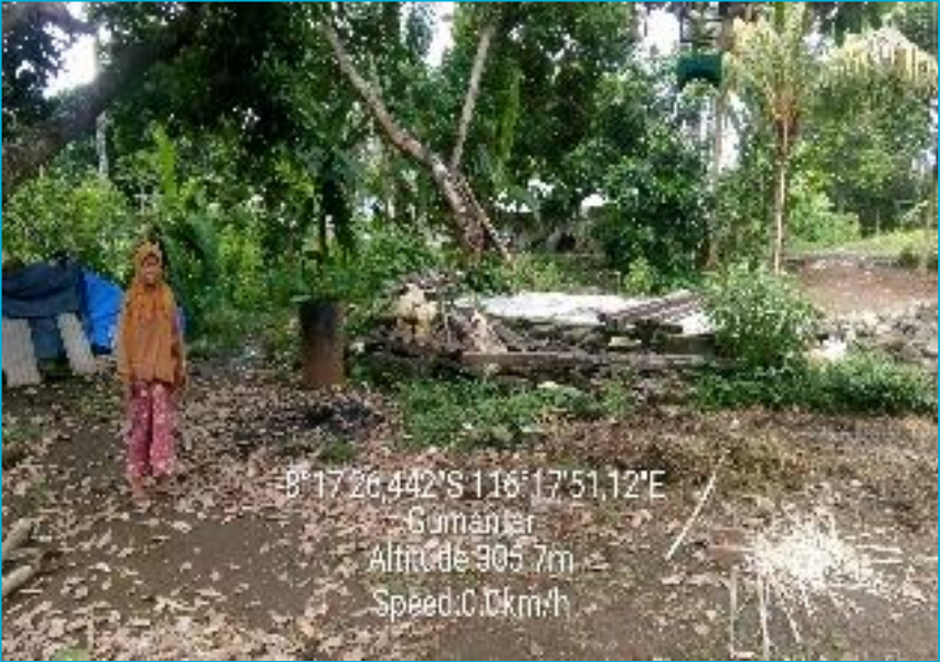
House condition BEFORE intervention
