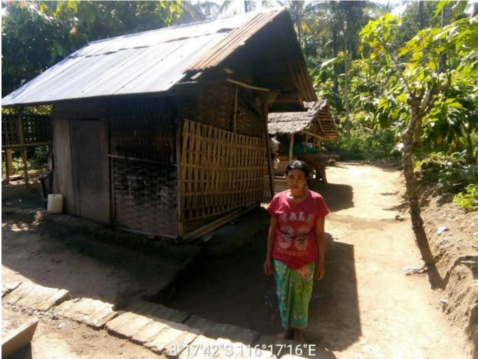
House condition BEFORE intervention
