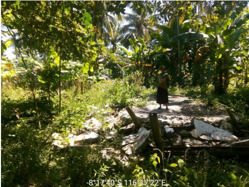
House condition BEFORE intervention
