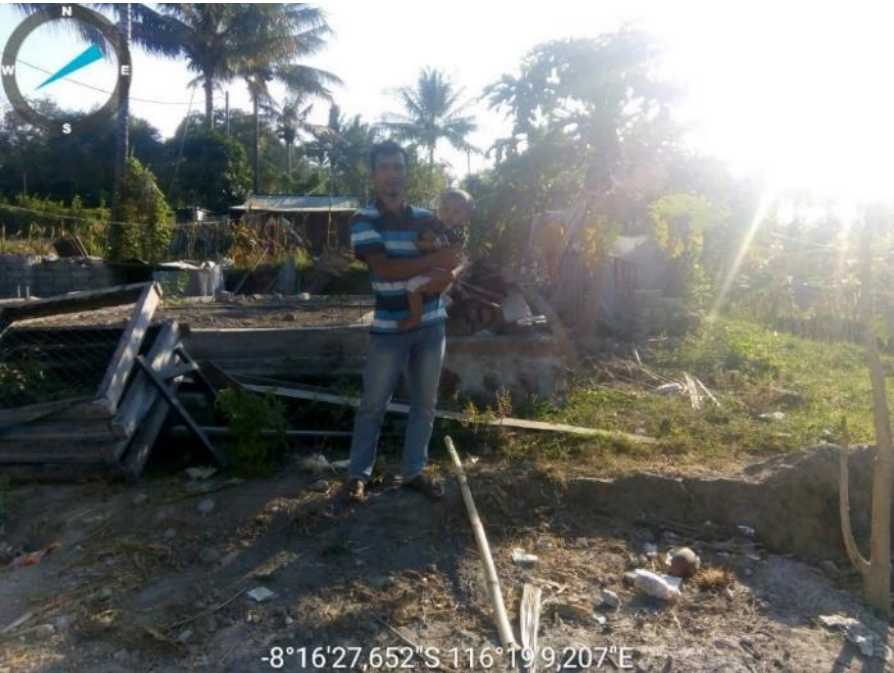
House condition BEFORE intervention
