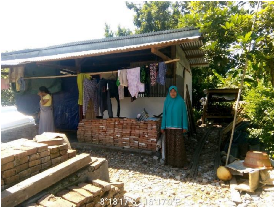
House condition BEFORE intervention
