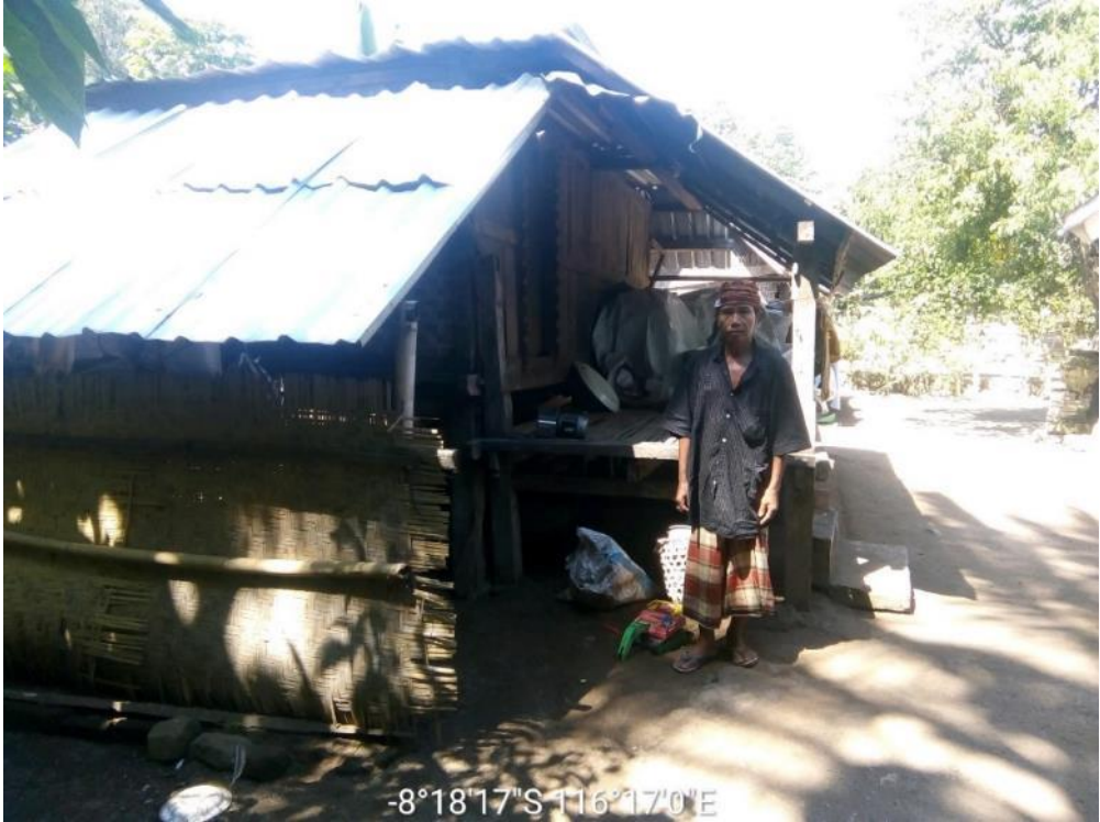
House condition BEFORE intervention
