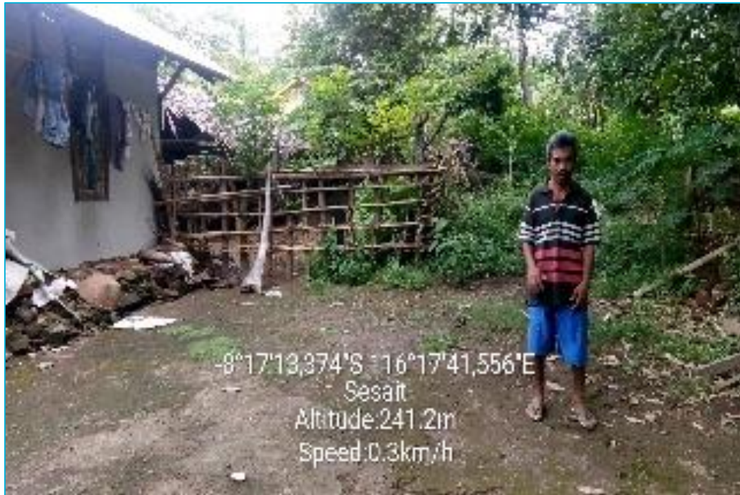
House condition BEFORE intervention
