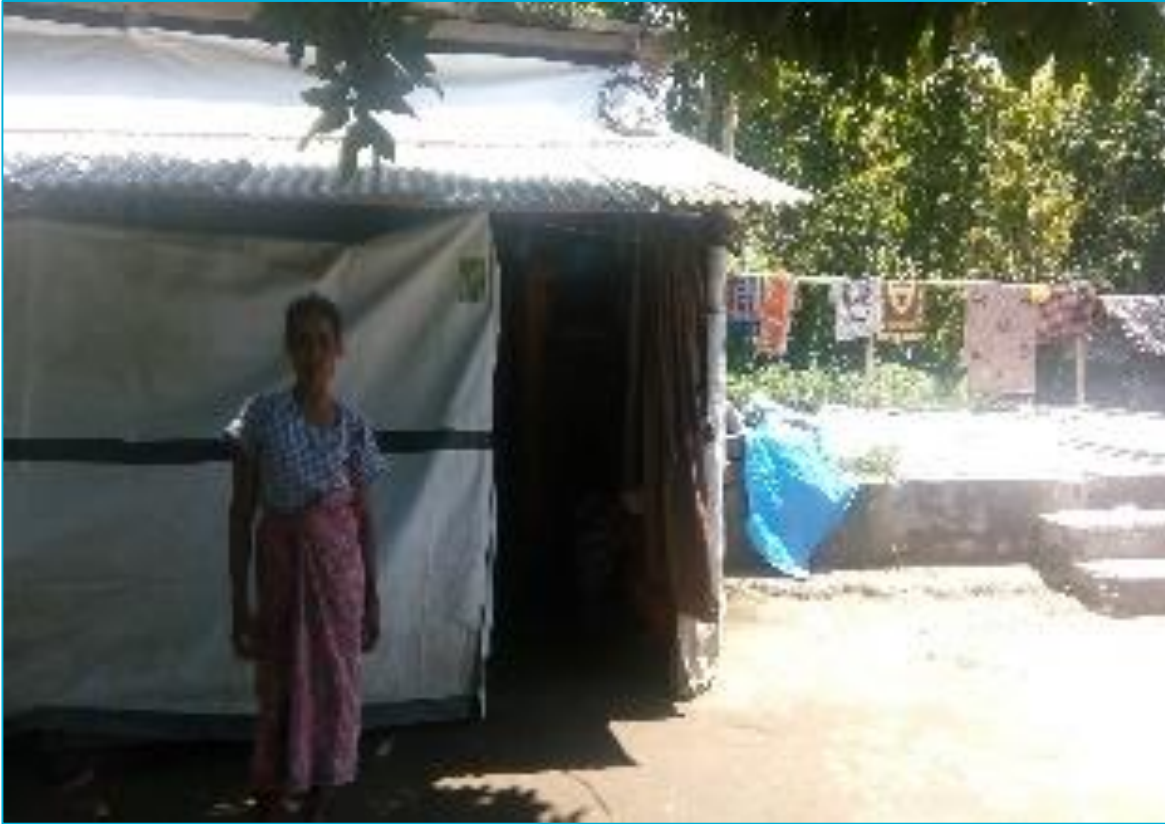
House condition BEFORE intervention
