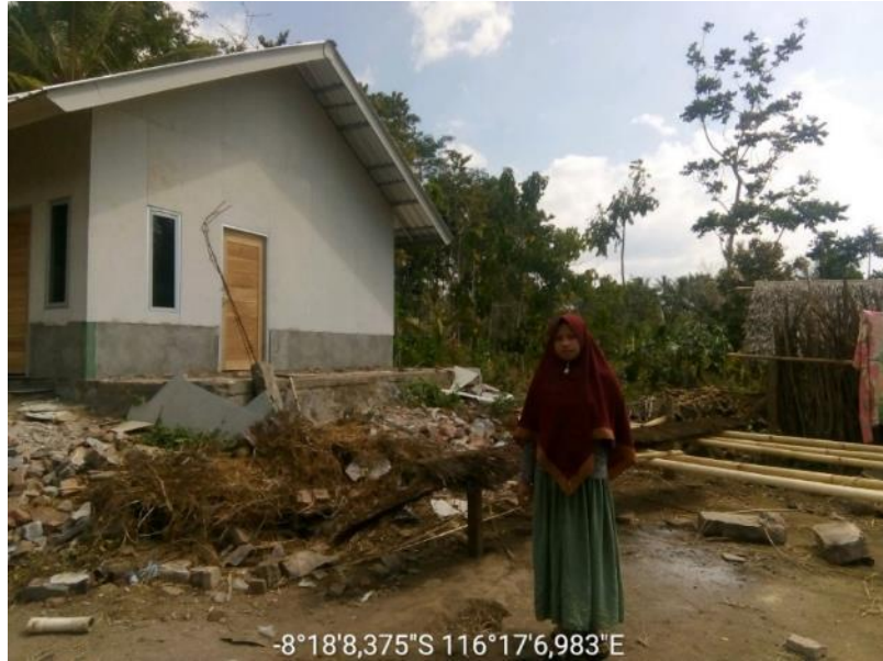
House condition BEFORE intervention
