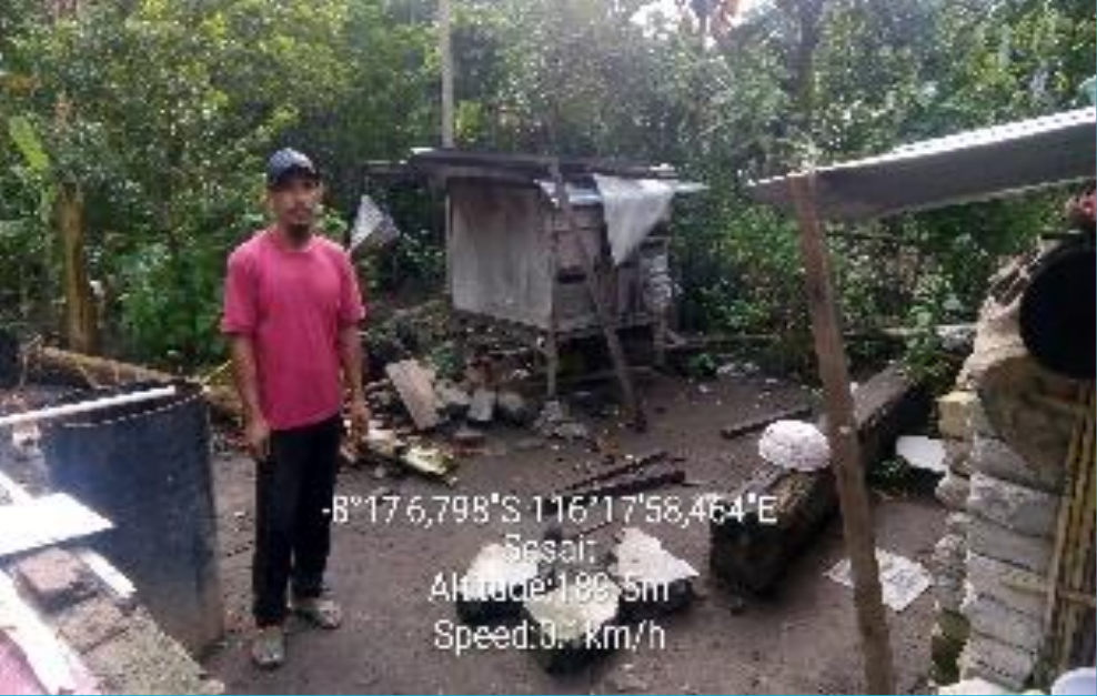
House condition BEFORE intervention
