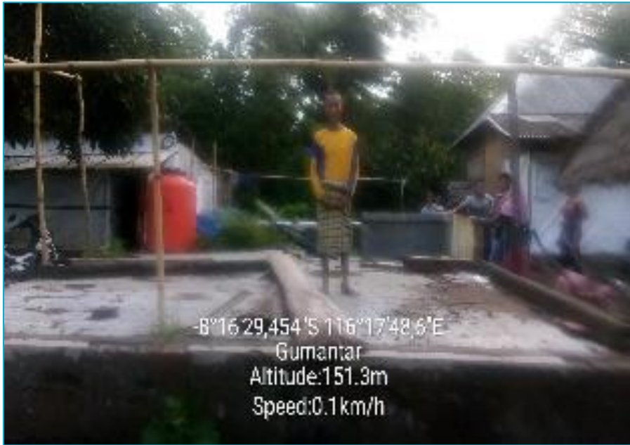
House condition BEFORE intervention
