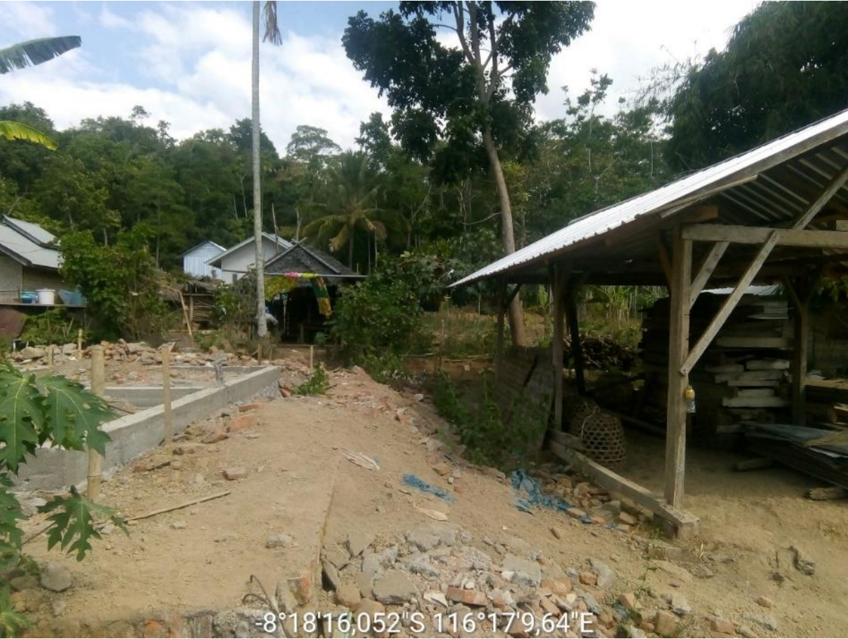
House condition BEFORE intervention
