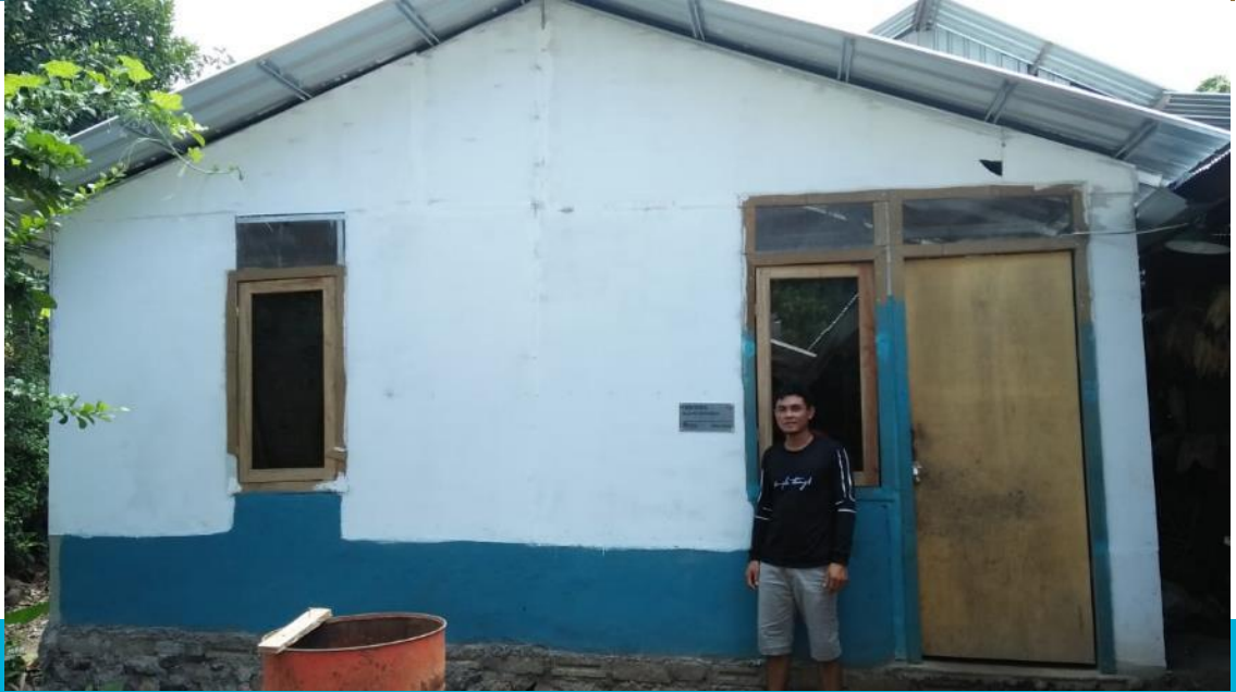
House condition AFTER intervention with temporary shelter assistance.
