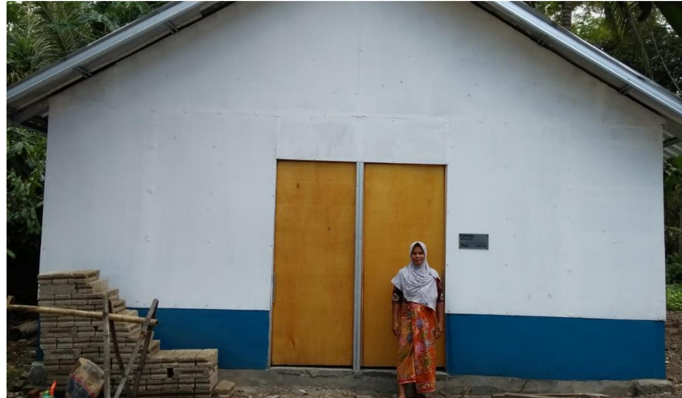
House condition AFTER intervention with temporary shelter assistance.
