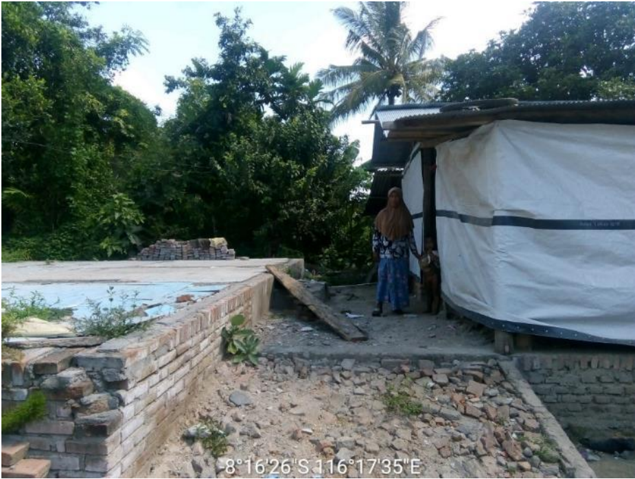
House condition BEFORE intervention
