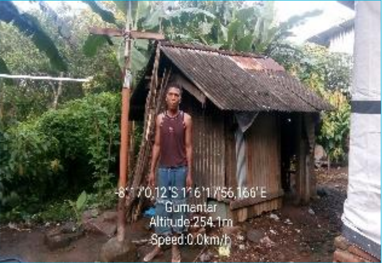
House condition BEFORE intervention
