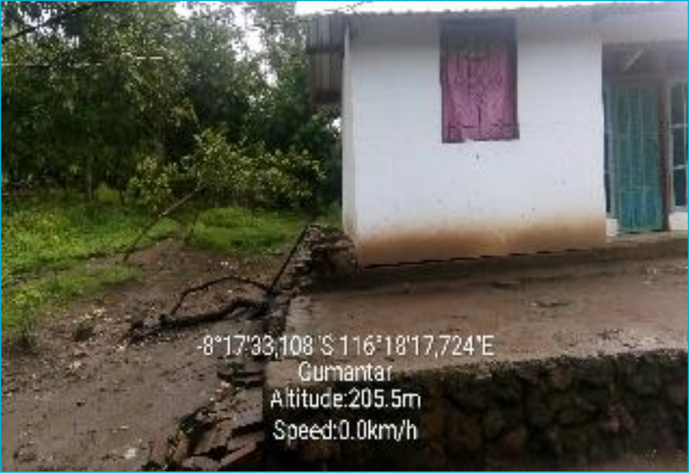
House condition BEFORE intervention
